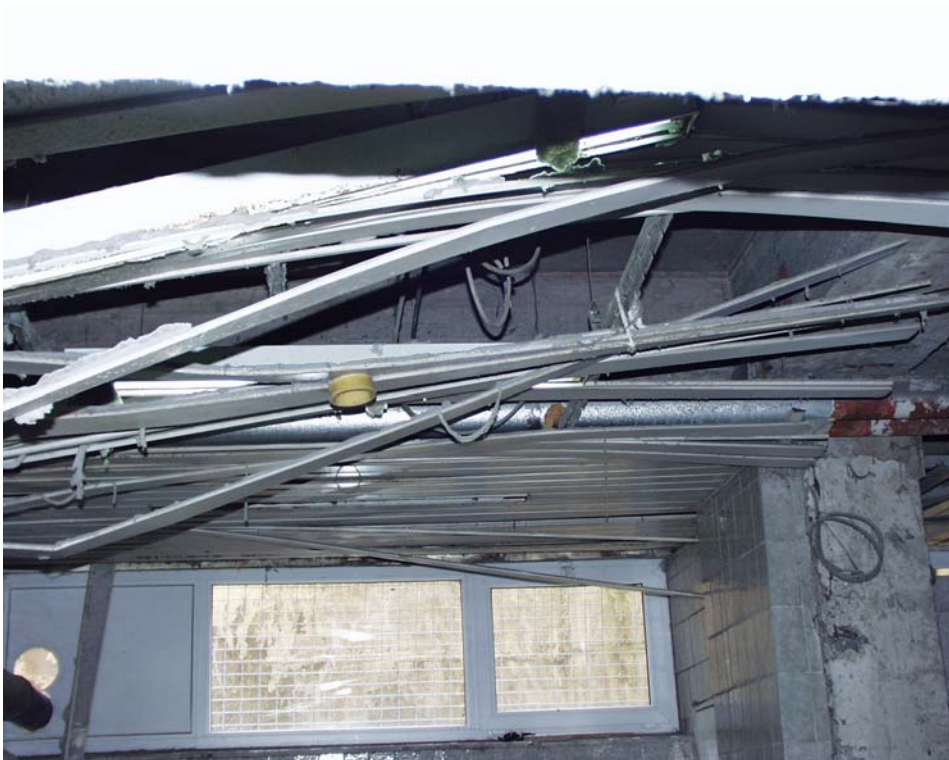
Suspended ceiling (basement)
