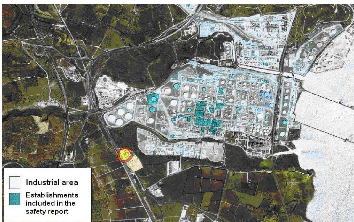
Fig. 33. ESSO tank farm in Augusta: accident scenario for a pool fire
