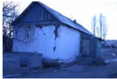
Picture 2. Seriously damaged house (outside and insight view) in Isakeev village. But it is evidently that the house was uninhabited long before earthquake
