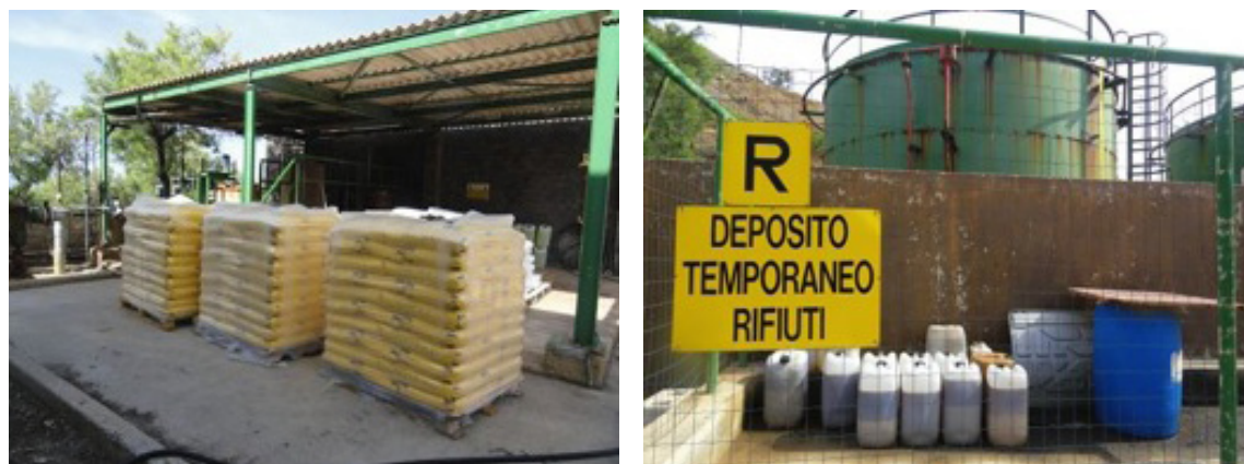
Fig. 16. Stocks of minerals and disinfectants and storage of waste oil at the Linosa desalination plant
