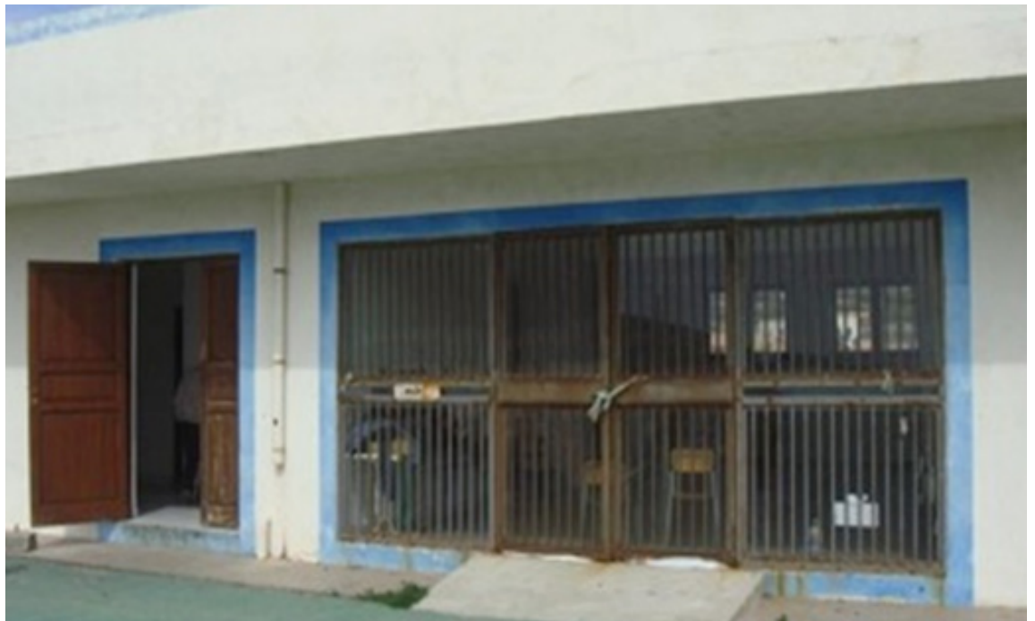
Fig. 10. Exterior and interior of Linosa Cultural Centre adapted to host migrants
