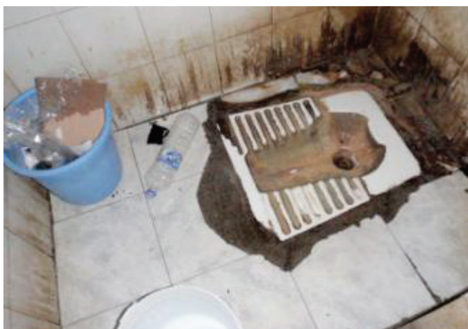
Figure 13: Toilet facility in one of the detention centres, April 2011
