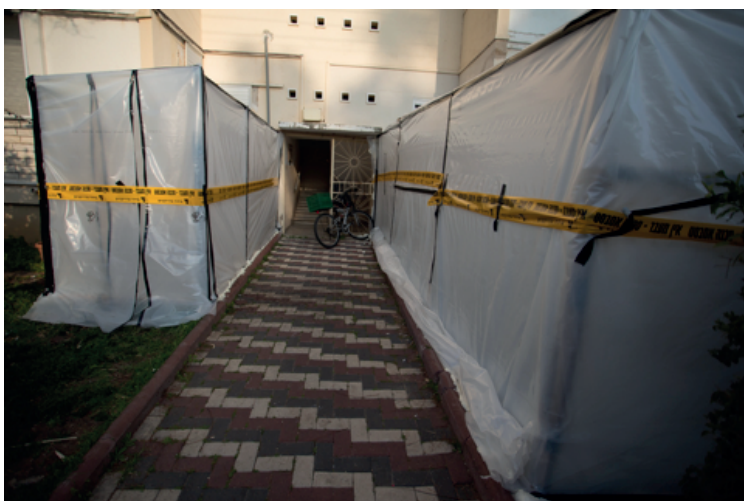
Figure 3: Asbestos clean-up project in Israel Source: Ministry of Environmental Protection
